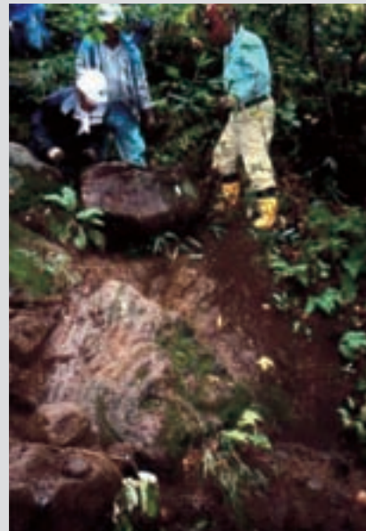
Maintenance of mountain trails using a nature-oriented construction method
